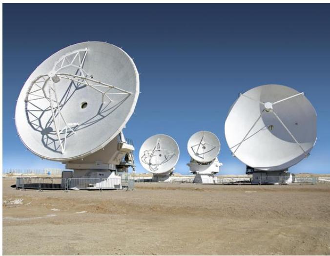
*The Atacama Desert is one of the driest places on Earth. This photomontage shows all four types of antennas that will be installed at the ALMA site: European, North American and Japanese 12-meter antennas, along with a 7-meter diameter one. Image courtesy ALMA (ESO/NAOJ/NRAO), W. Garnier (ALMA).*
